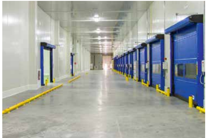
Guardrails for aisle
