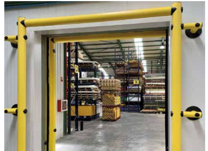
Guardrails for aisle
