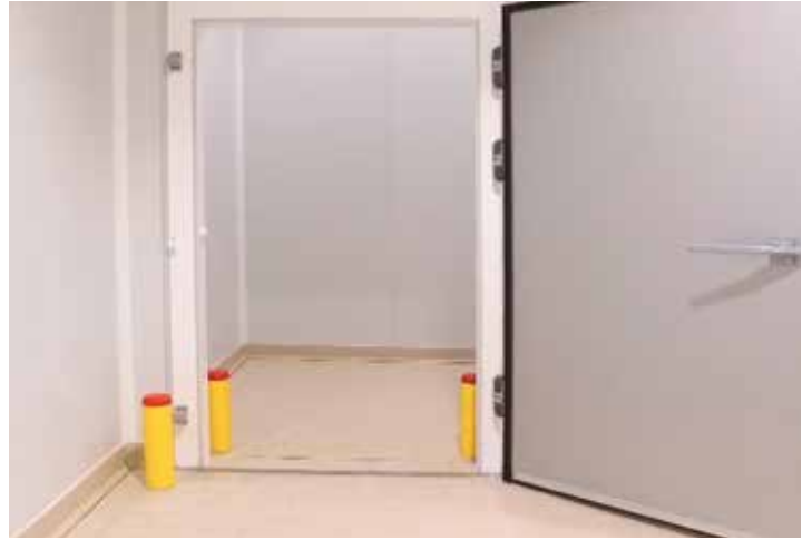
Bollards for protection of shelves and doors
